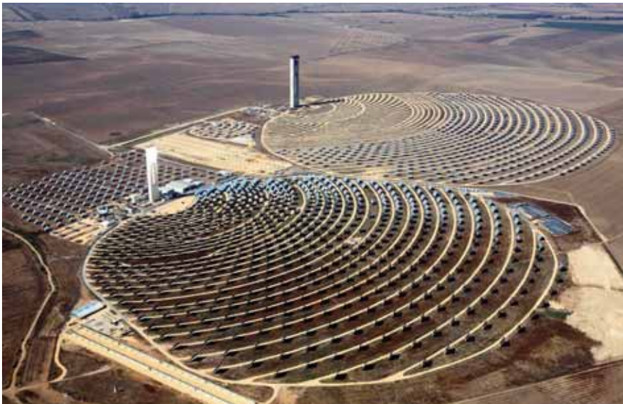
The PS10 power tower CSP plant (foreground) and the PS20, Sanlúcar la Mayor, near Seville, Spain.
